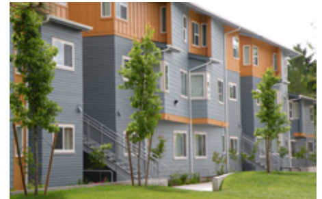
Villa de San Juan Bautista | Farmworker Housing
