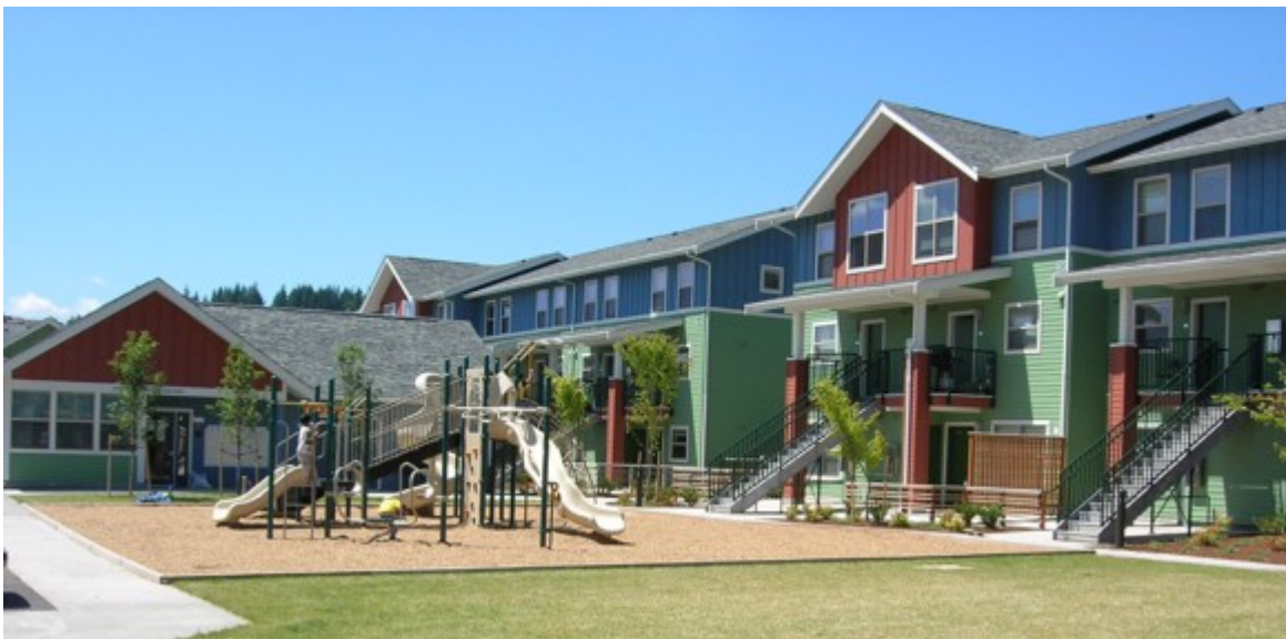
La Casa de la Familia Santa: a CHS property providing 45 units of affordable housing for farmworkers and their families in Centralia
